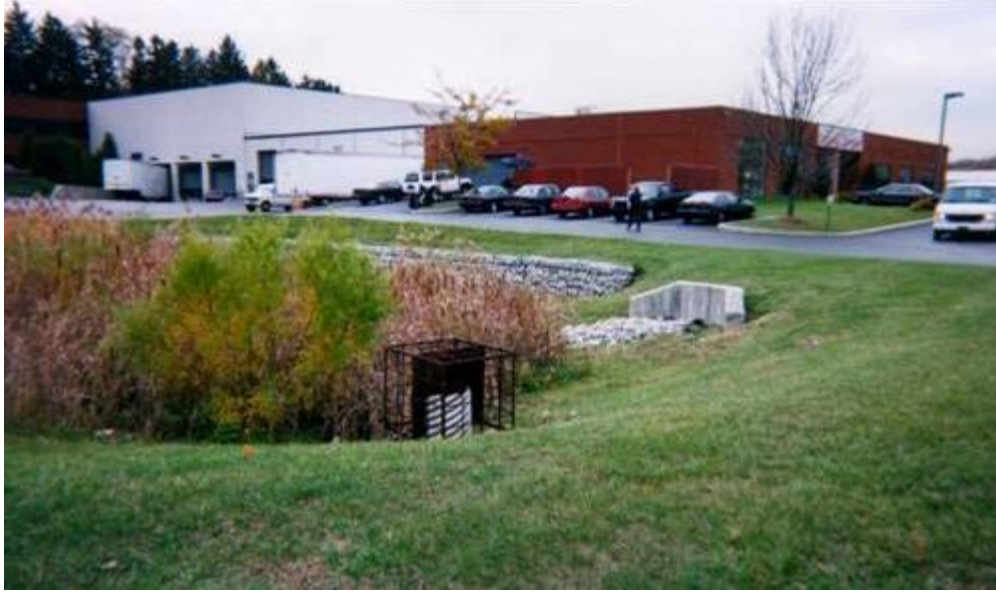
FIGURE 4-29 Dry Extended Detention Basin with Shallow Marsh
