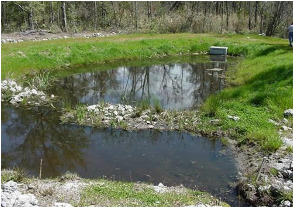
FIGURE 4-8 Permanent Pool of Water in Wet Detention Basin
