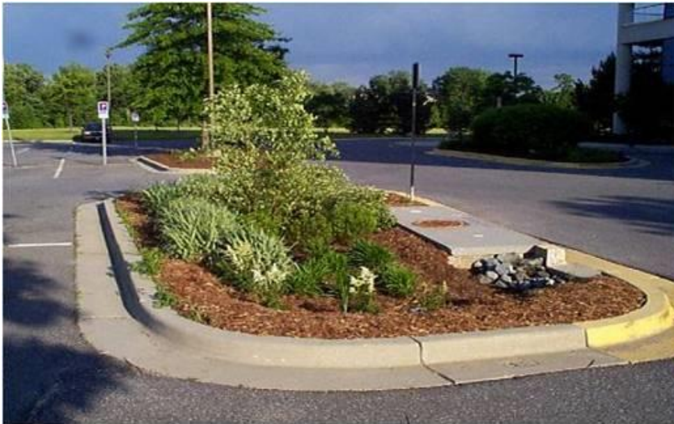
FIGURE 4-3 Bioretention in Parking Lot Island
