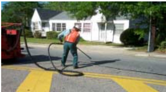
Crack-sealing to extend the life of street surfaces
